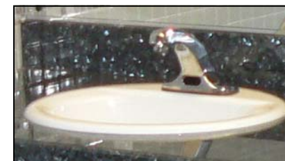
Water Efficient Sink Fixtures
